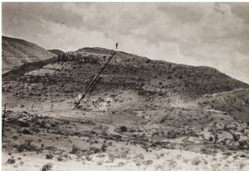
Figure 11. North part of Blanchard mine area. Adit on fault zone (f) Council Spring limestone (columnar limestone) against lower part of Story formation and an alteration zone above the Council Spring limestone along road cut.
